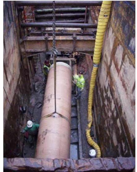
*Installation of a new multi-million dollar 42" sanitary sewer interceptor was completed in the summer of 2012.*
